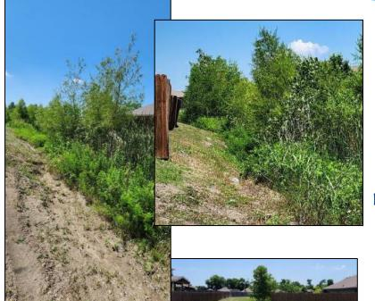
Unfortunately, over the years the swell walls have eroded away causing the earth to slowly begin settling back into the ravine. This erosion is a direct result of the irrigation system not being maintained which allowed the root systems to die, which allowed the earth to erode. This erosion has begun to pull the private property fences and soil into the ravine as the earth continues to shift from the failed ravine.
